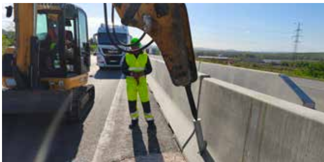
M1 near Bicske (Hungary): From zero to 60 km of concrete safety barriers in a year!
