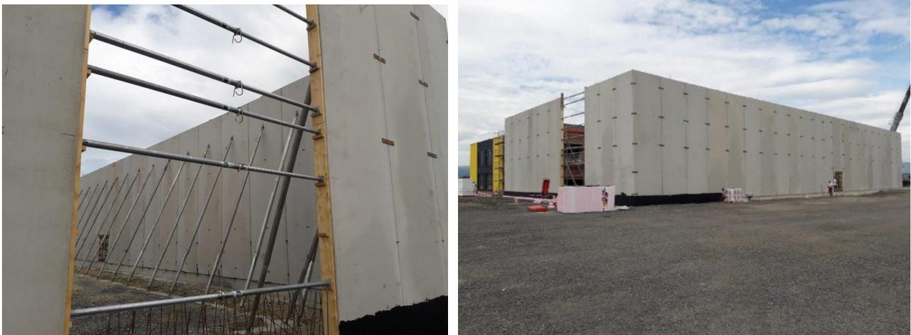
**Innovative technology and quality:** The precast concrete parts come from Kammel and were assembled on site with the highest precision and poured with in-situ concrete. Reprint free of charge with attribution: © Kirchdorfer
